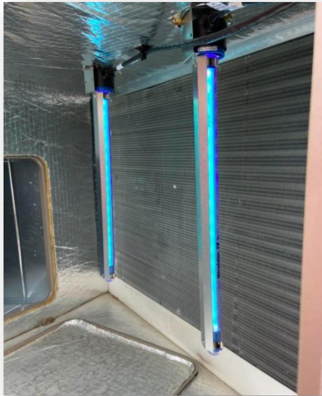
Dual Compact-Series shown in in a package unit using magnetic mount and shields.
